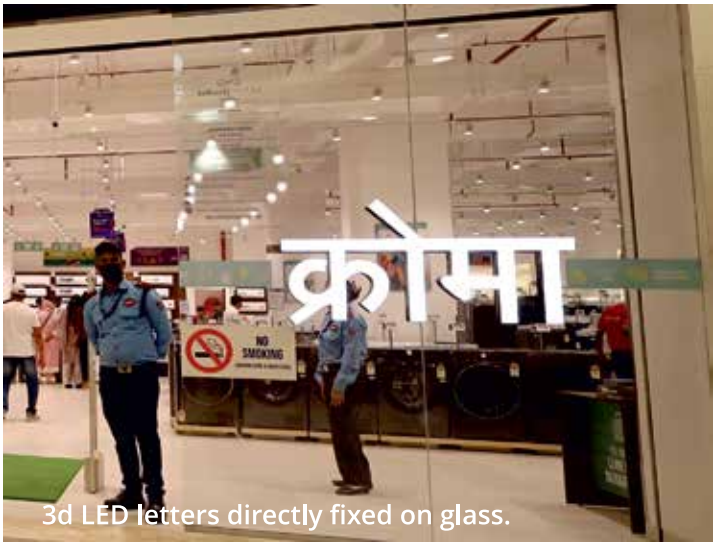
3d LED letters directly fixed on glass.
